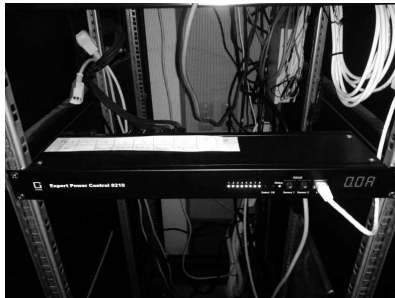
Fig. 3. Computer controlled power switch Expert Power Control 8210
